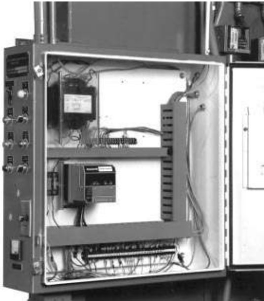
Fig. 7. Electrical panel installation.
